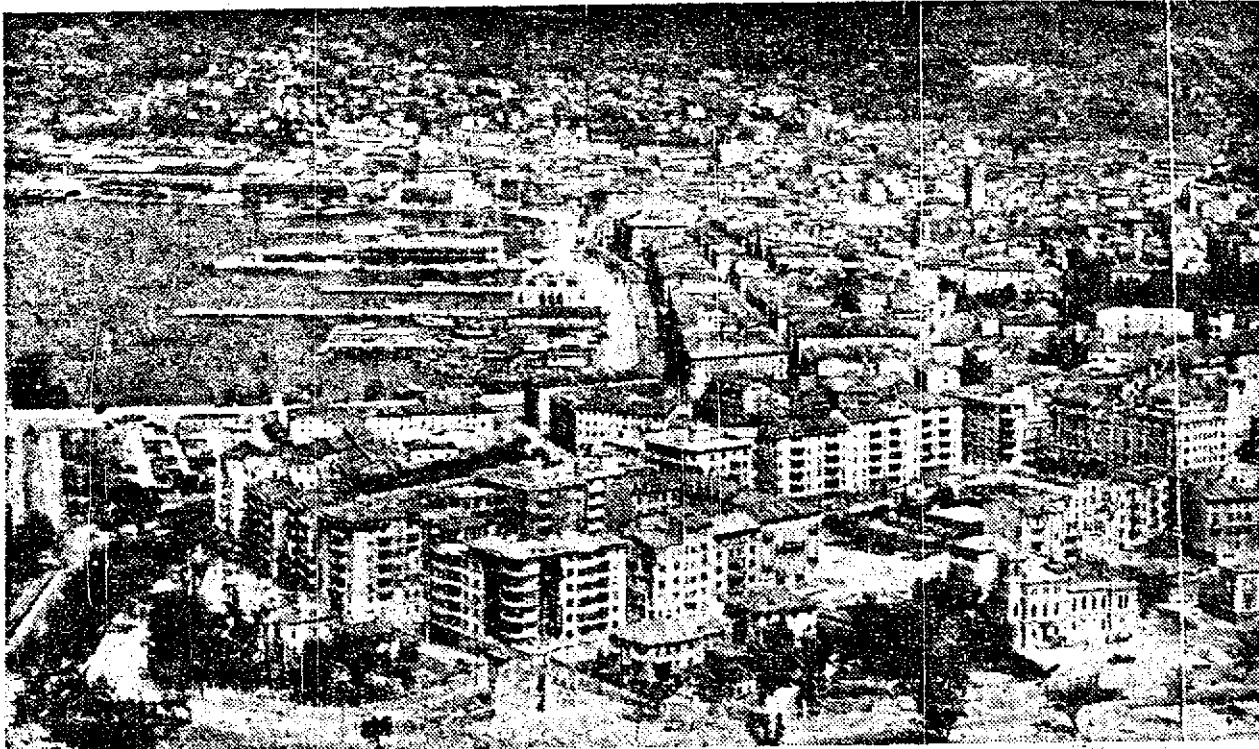
This is an airview of the city of Trieste. The view is looking northeast with rail yards at the lower left and apartment buildings lower center. Part of the Trieste harbor is at the upper left. —Acme
